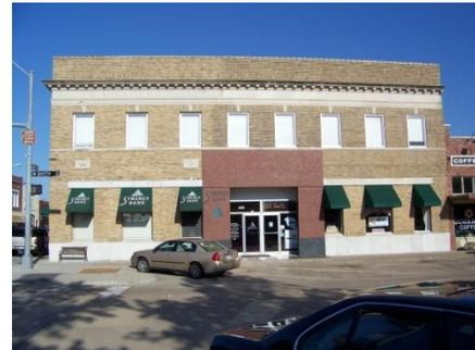
The façade was re-designed, un-matched floor levels between the two buildings were connected, windows changed and a central entrance was created on 6th Street. A drive-through banking window was installed at the rear of the building as part of a large one-story addition. 603-605 Main Street was renovated at the same time; the brick on its façade matches that of the 1954 façade. More recently, the Synergy Bank has occupied the building with one tenant on the ground floor.
