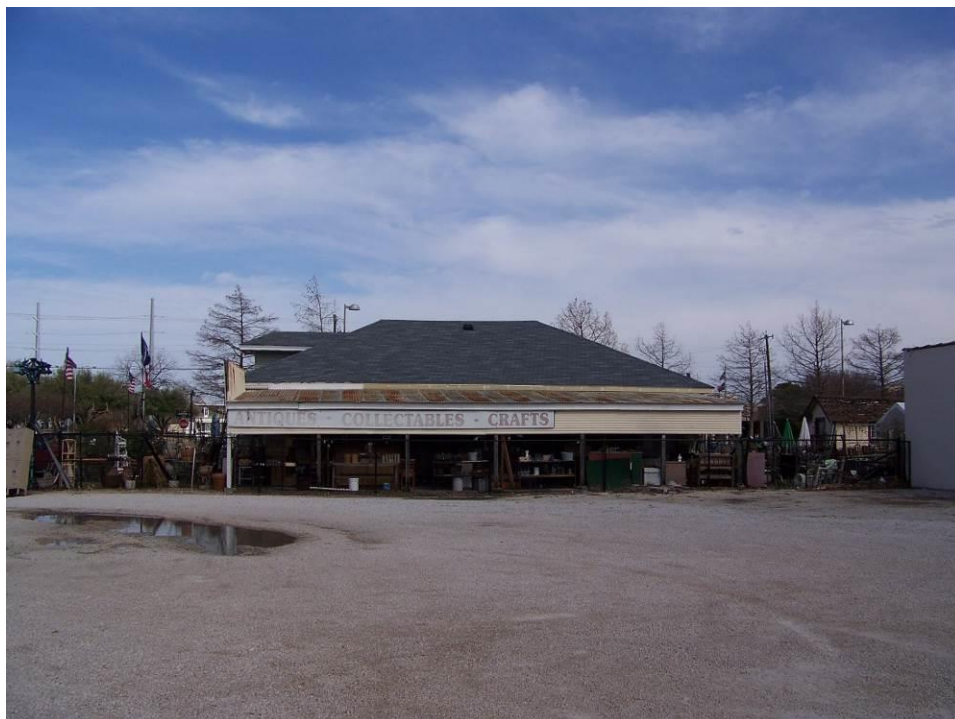
Photo 3: View north from gravel parking lot of south elevation of house. Camera facing north.
