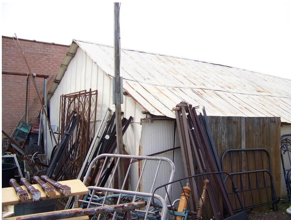
Photo 6: View southwest of partial east and north elevation of garage. Camera facing southwest.
