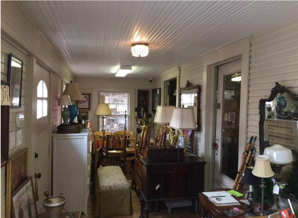
Photo 9: Interior view of enclosed front porch. Note the wood siding, front door and window trim of the original front elevation on the right side of photograph. Camera facing north.
