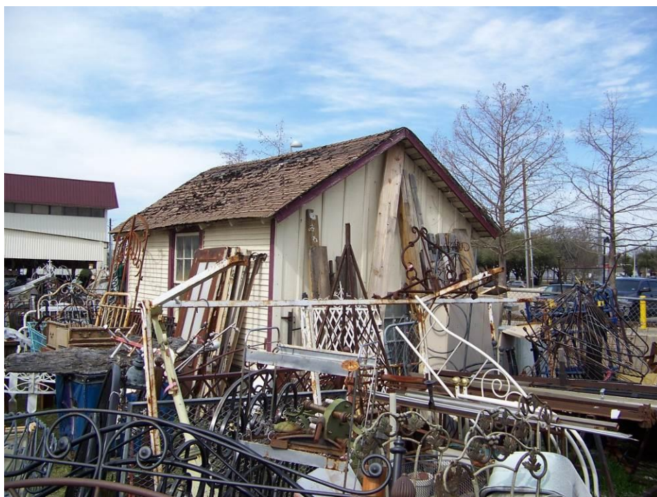
Photo 8: View of bedroom structure. Camera facing northwest.
