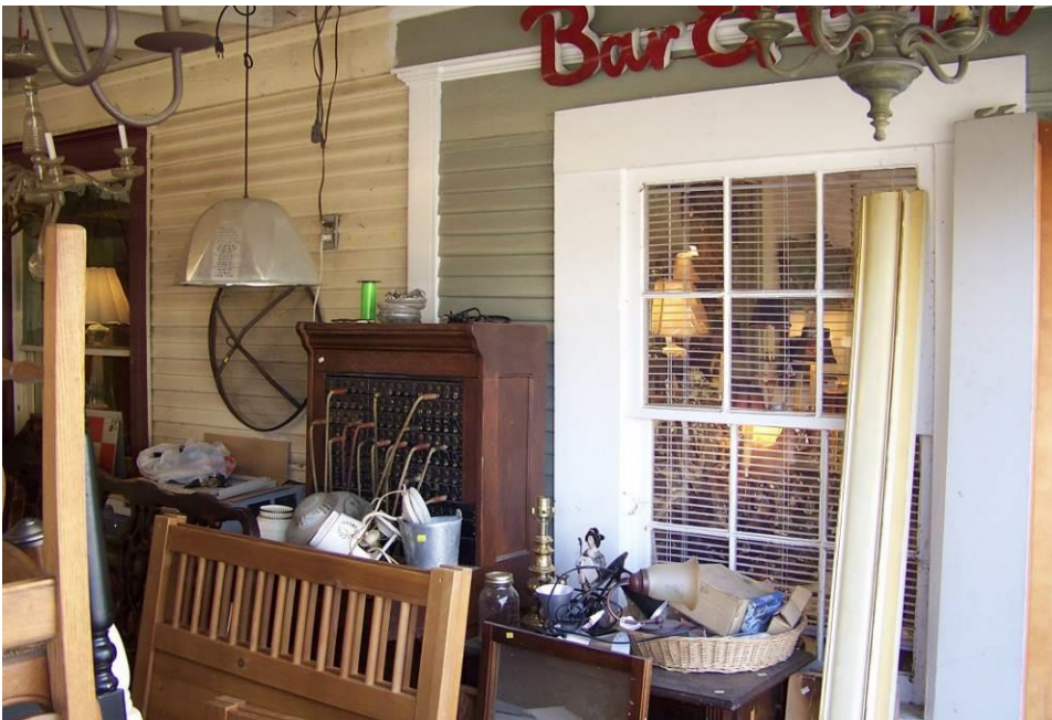
Photo 10: View of north porch enclosure wall painted green paint. The original window installed at this location at time of enclosure was used to replace deteriorated front window. This window is from a salvage yard and selected because it matched original. Camera facing southeast.
