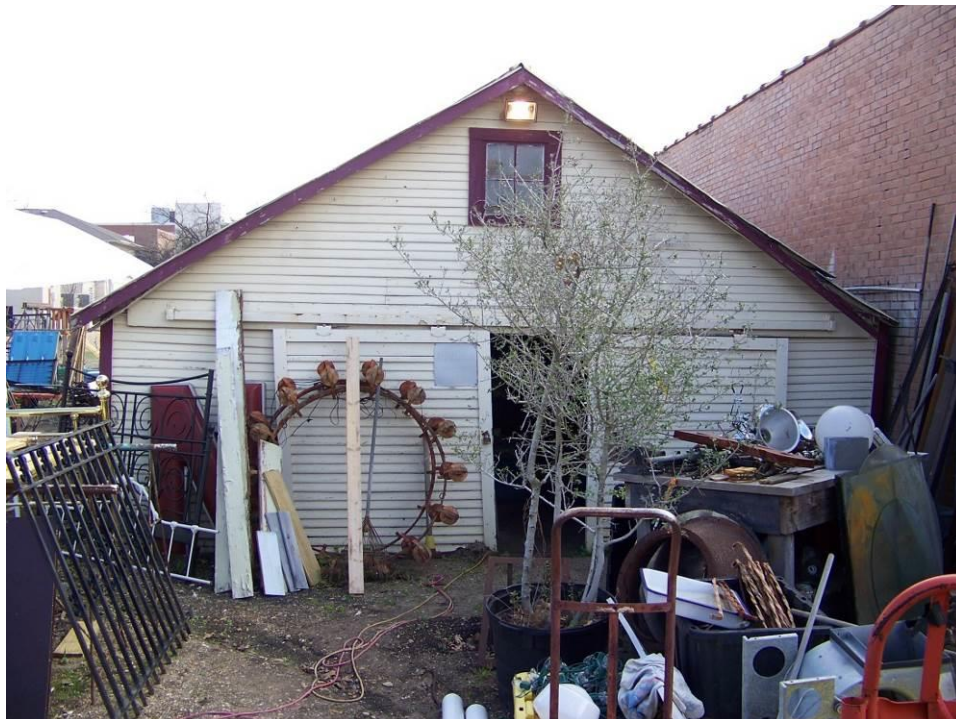
Photo 5: View east from backyard of west elevation of garage. Camera facing east.
