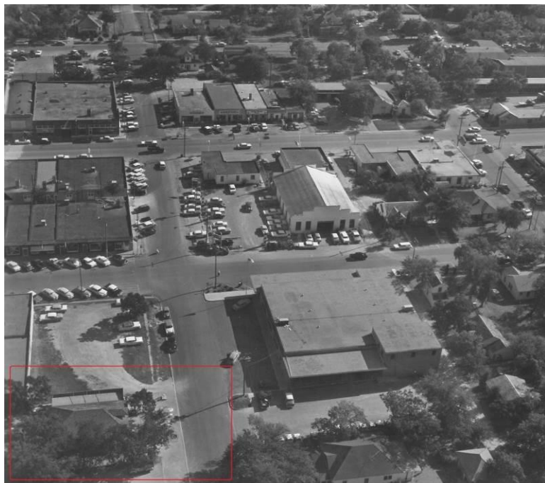
Figure 8: View looking southwest toward 212 N. 7 th Street, marked in red. Note the shed constructed the length of the south elevation, c 1958. Courtesy of the Garland Landmark Society.
